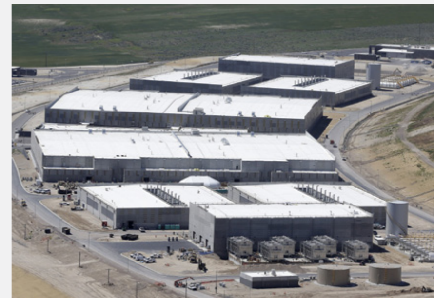
US NSA Data Center (photo as of 2013)
